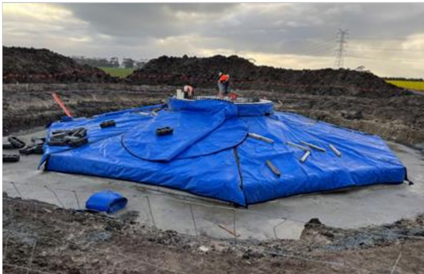
Plate 16: Footing covered with thermal blankets - Berrybank Windfarm Stage 2 - icubed consulting
