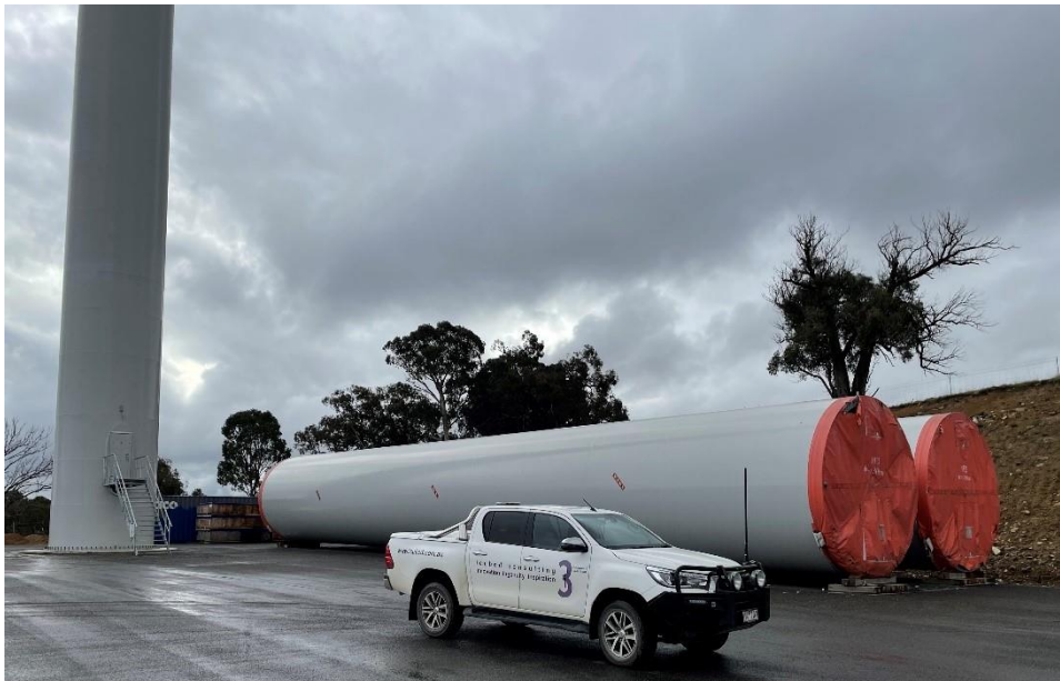
Plate 7: Tower Components – Bango Windfarm, NSW
