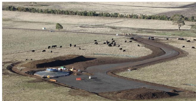
Plate 5: Component and Erection Hardstand – Mt Mercer Windfarm, Victoria
