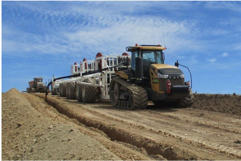
Plate 2: 33kV MV Power Cable - Crudine Ridge Wind Farm, NSW
