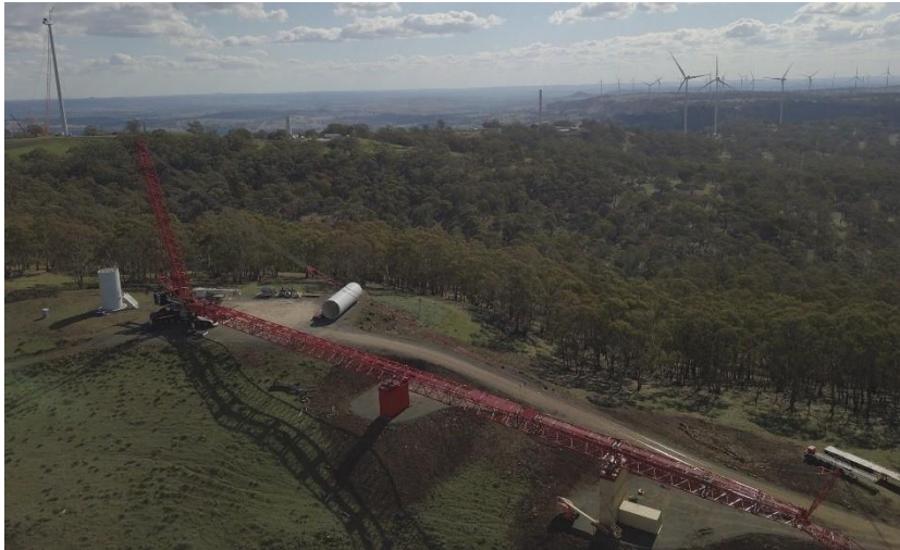
Plate 9: Main Crane Assembly – Sapphire Windfarm, NSW
