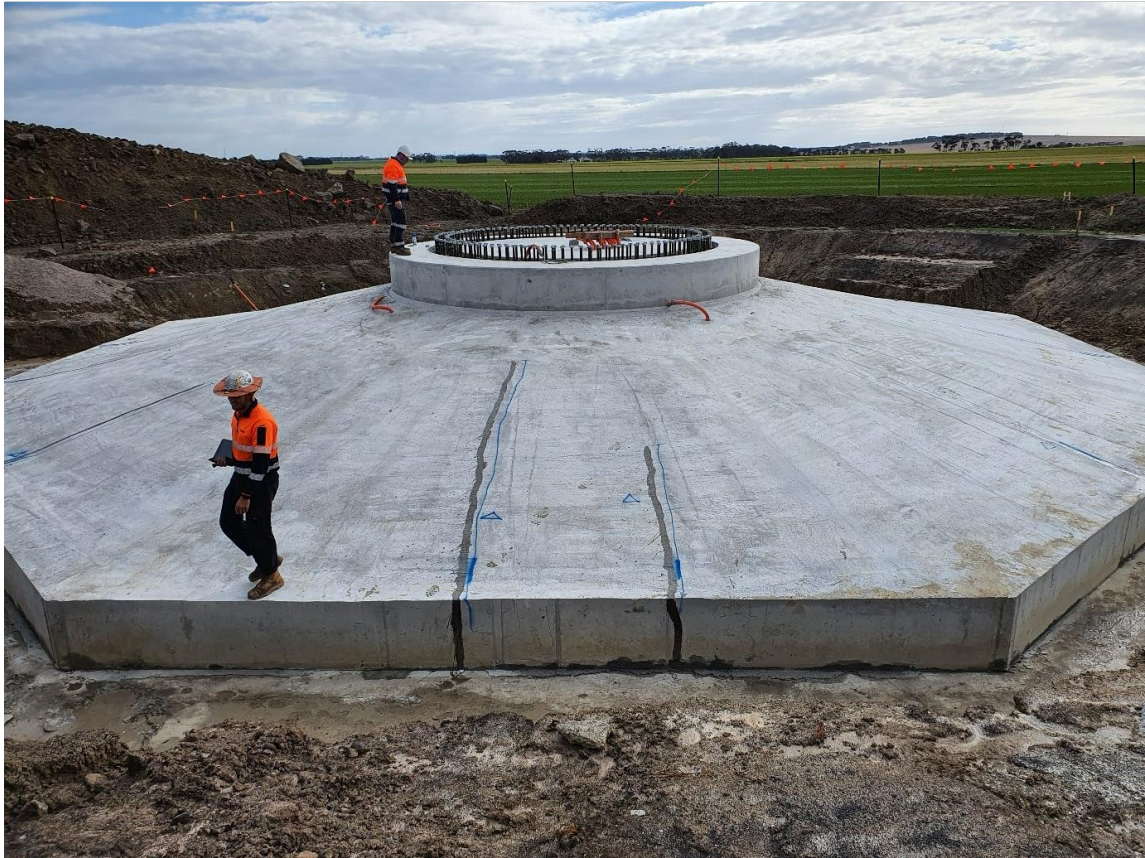
Plate 12: Thermal differential cracks repaired - Berrybank Windfarm Stage 2 - icubed consulting
