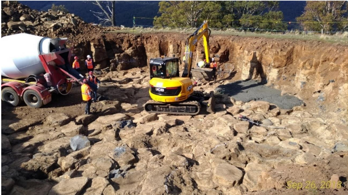
Plate 11: Example footing requiring 'dental' flowable fill – Cattle Hill Wind Farm.
