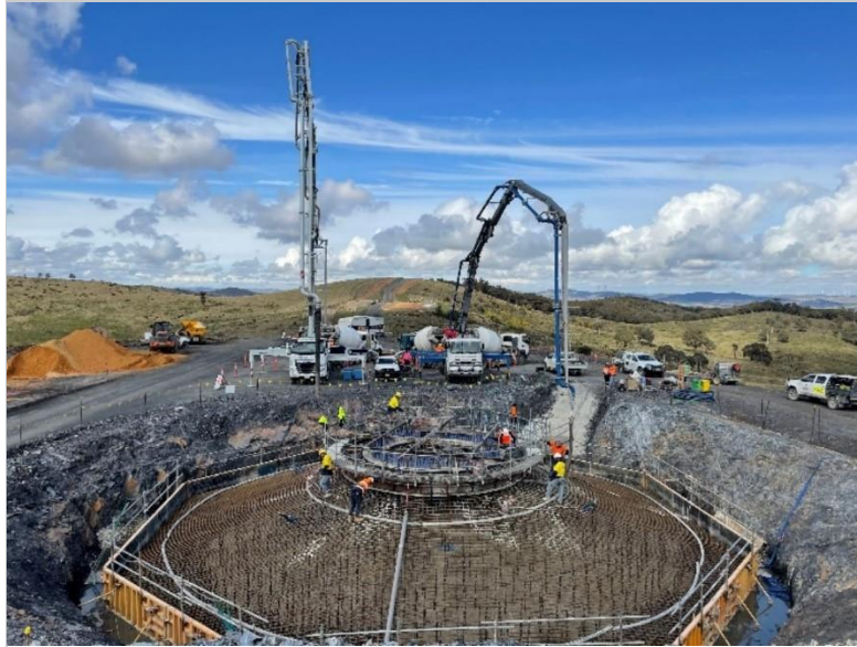
Plate 6: Gravity Footing – Rye Park Windfarm, Victoria
