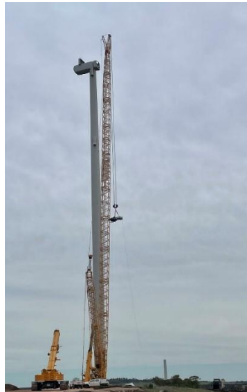
Plate 10: Main Crane Operating – Dulacca Windfarm, Queensland
