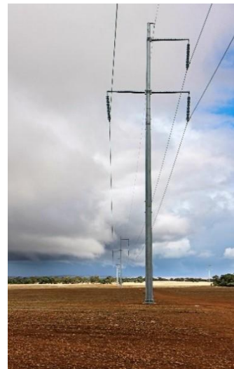
Plate 3: 275kV Overhead
