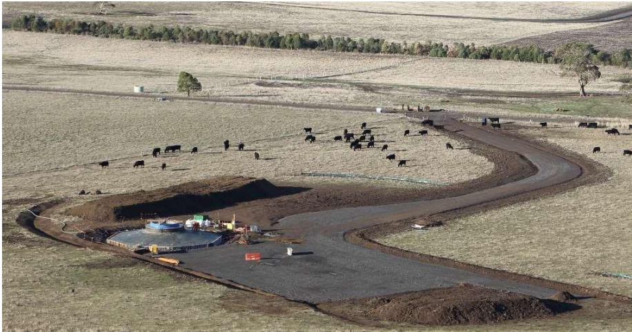
Plate 6: Component and Erection Hardstand – Mt Mercer Windfarm, Victoria
