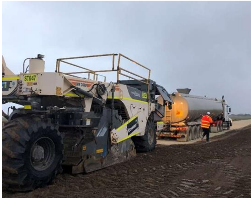
Plate 25: Subgrade Stabilisation, Murra Warra Windfarm, Victoria
