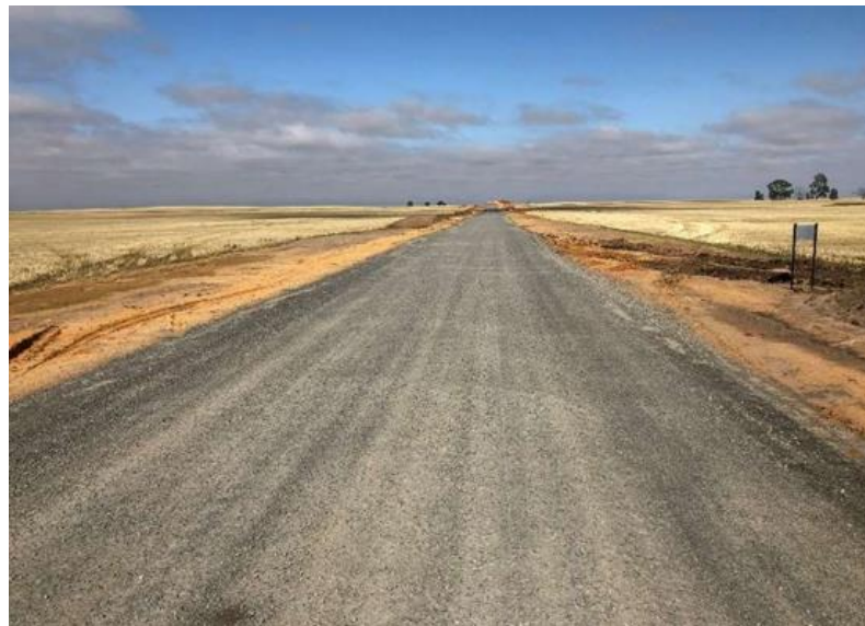
Plate 26: Completed Pavement, Murra Warra Windfarm, Victoria
