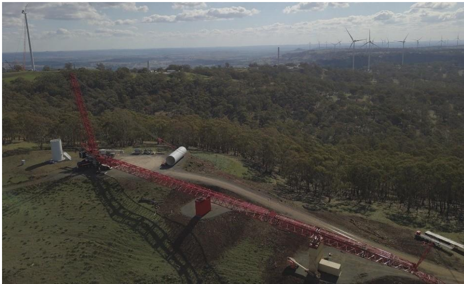
Plate 9: Main Crane Assembly – Sapphire Windfarm, NSW
