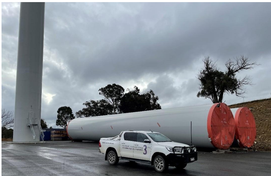
Plate 7: Tower Components – Bango Windfarm, NSW
