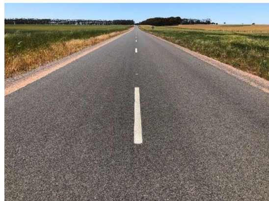
Plate 19: After - Woomdoo-Streatham Road, Dundonnell Windfarm, Victoria
