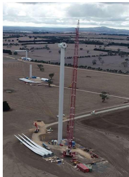
Plate 10: Main Crane Operating – Moorabool Windfarm, Victoria
