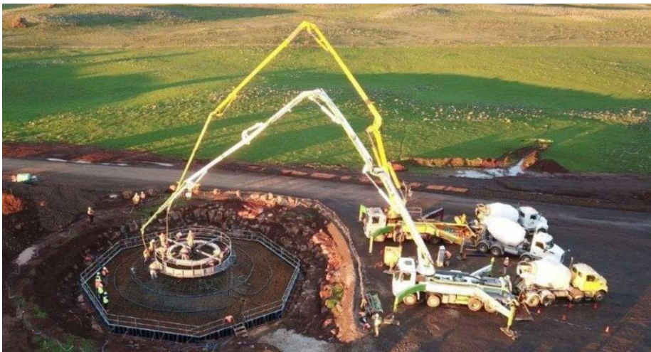
Plate 5: Gravity Foundation – Dundonnell Windfarm, Victoria
