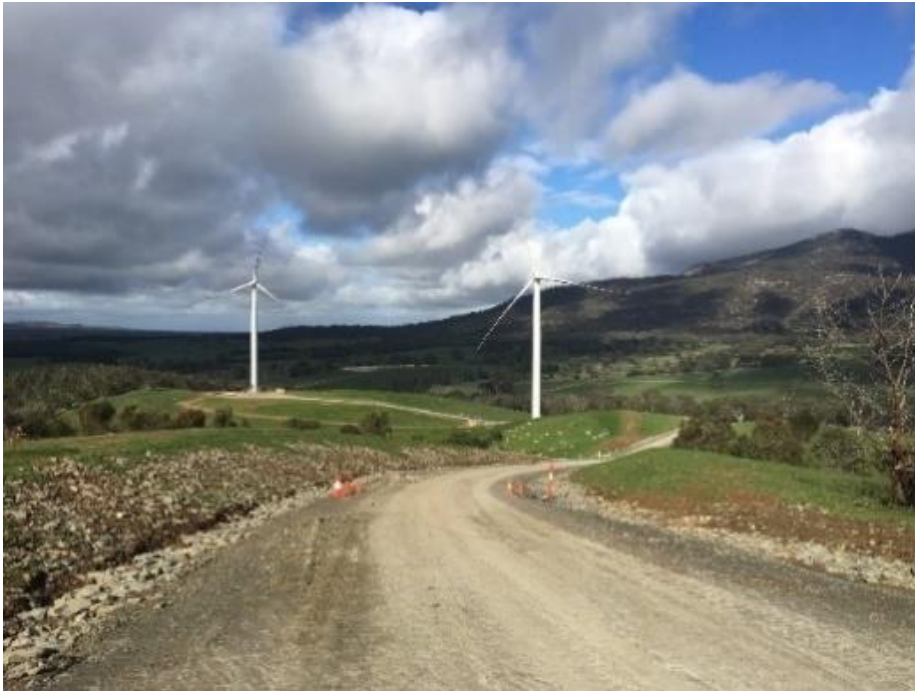
Plate 4: Typical Track – Ararat Windfarm, Victoria
