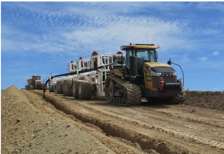
Plate 2: 33kV MV Power Cable - Crudine Ridge Wind Farm, NSW
